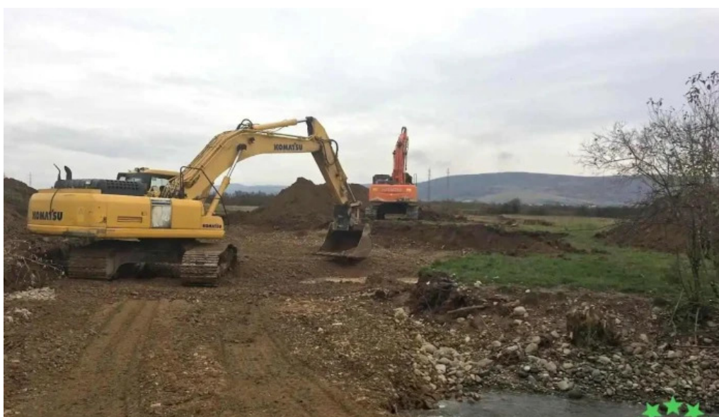
Beton construct s r l ale?d
